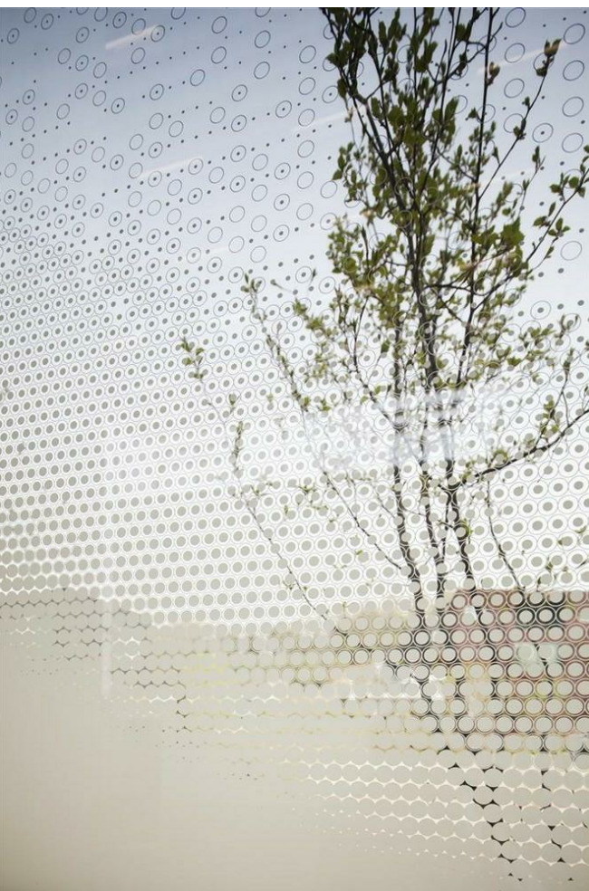
BL-02 GLASS BALUSTRADE Material: Framed glass Finish: Fritted Glass
